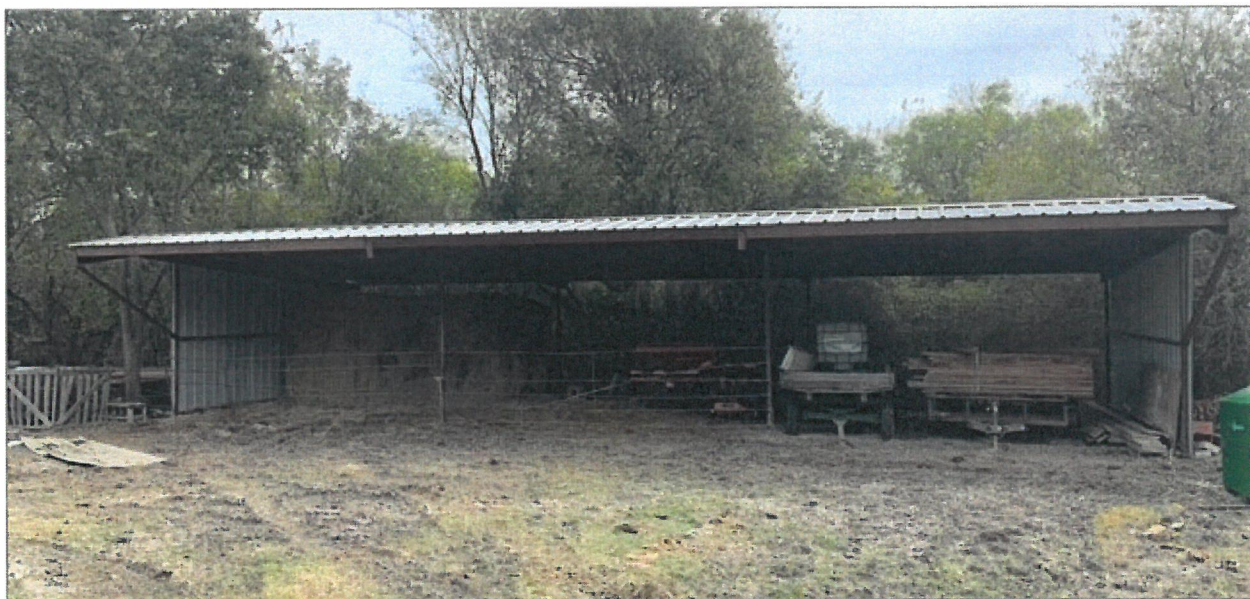
BUILDING #3: AGRICULTURAL ACCESSORY BUILDING SITUATED WITHIN THE 100-YEAR FLOODPLAIN
