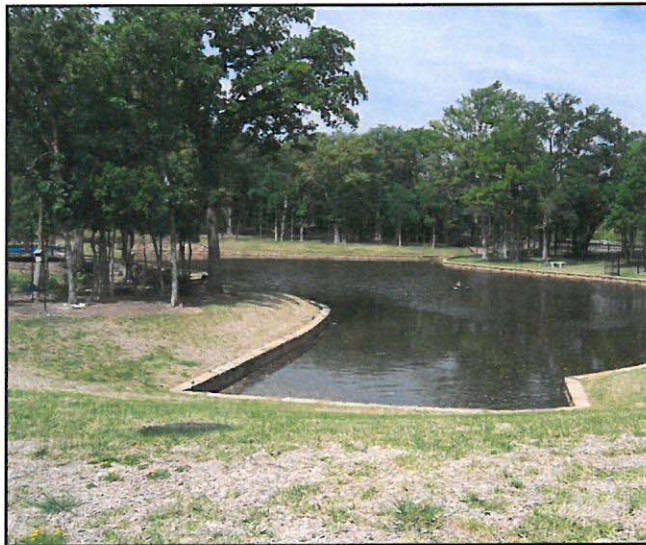
Figure 1: Retention Pond with Hardedge.
