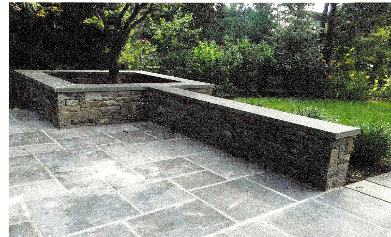
TRAIL HEAD REST STATION STONE SEAT WALL AND RAISED PLANTER EXAMPLE PHOTO
