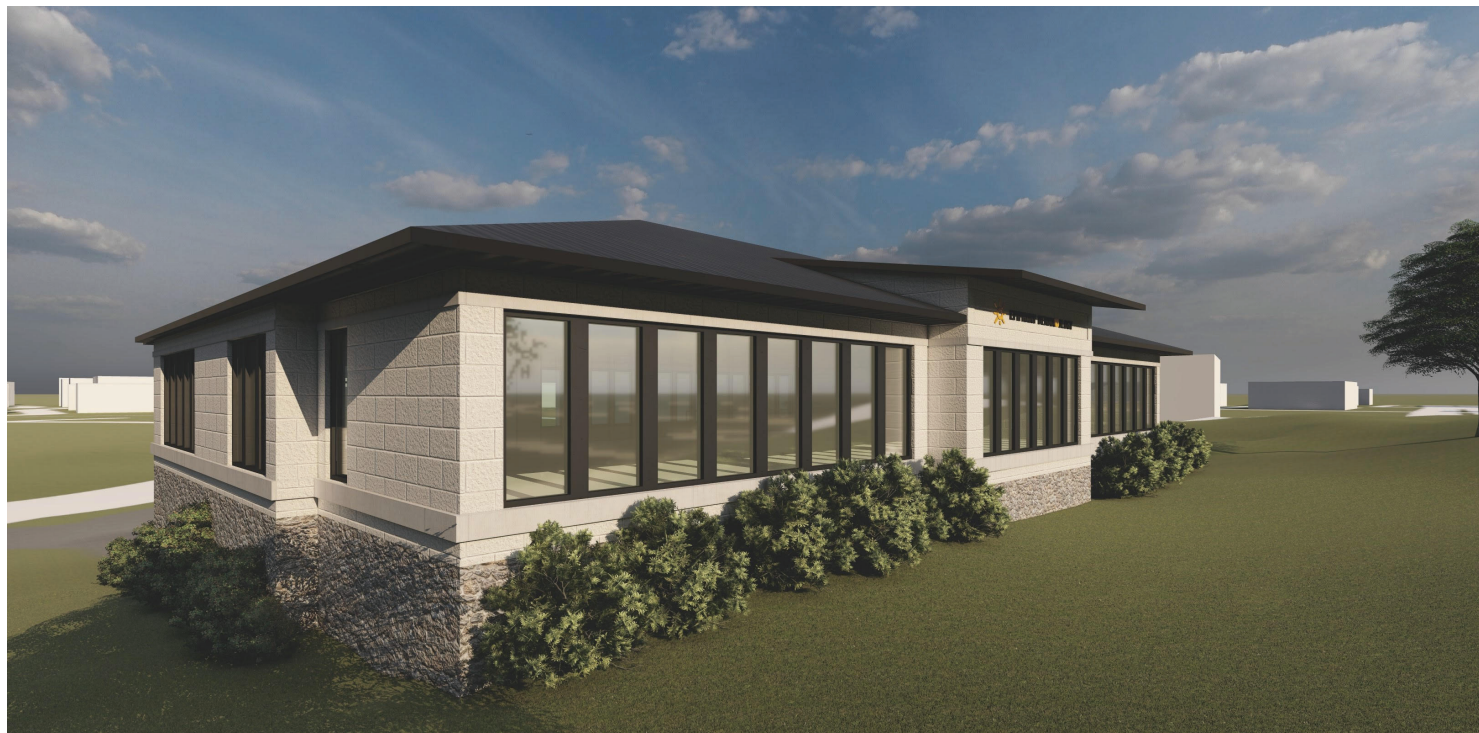
VIEW VISIBLE FROM RIDGE RD, EASTERN FACADE
