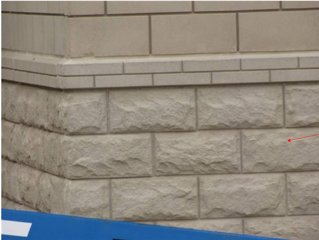
PHOTO IMAGE CLOSE-UP VIEW OF PREVIOUS INSTALLATION OF FORM LINER #892
