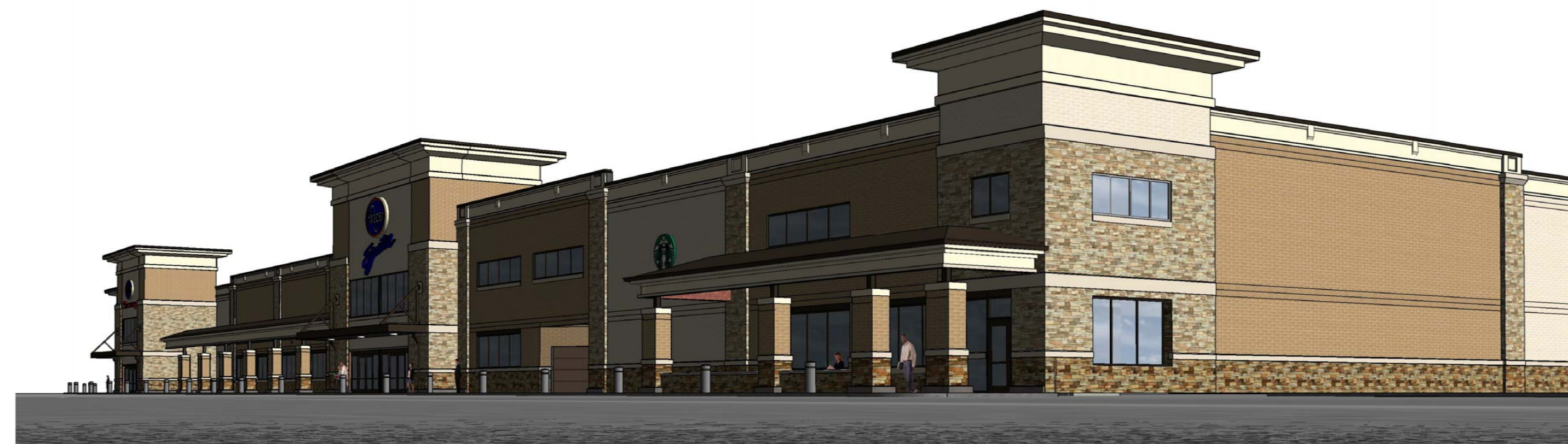
3 VIEW FROM MEMORIAL DRIVE
