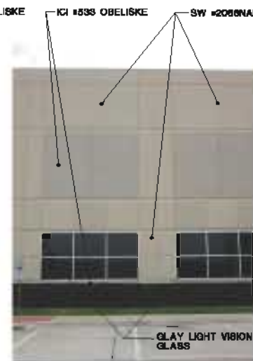
TYPICAL CONC. TILT PANEL WITH VISION GLASS
