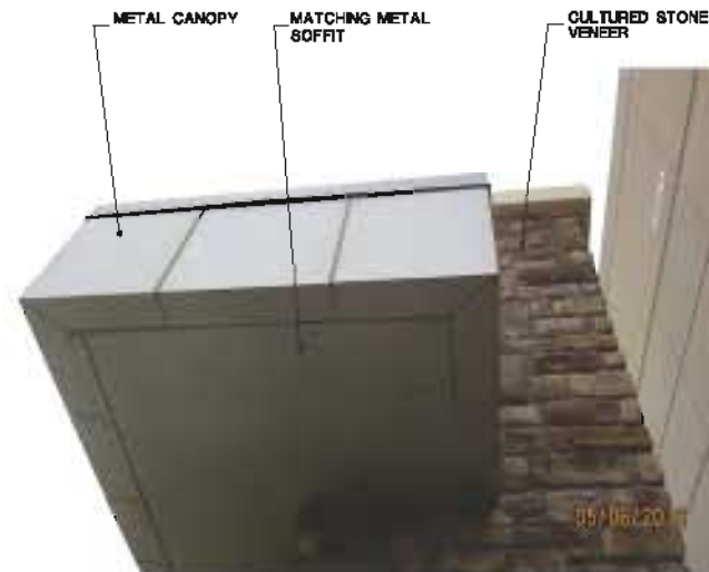
METAL CANOPY AT OFFICE ENTRY AREA
