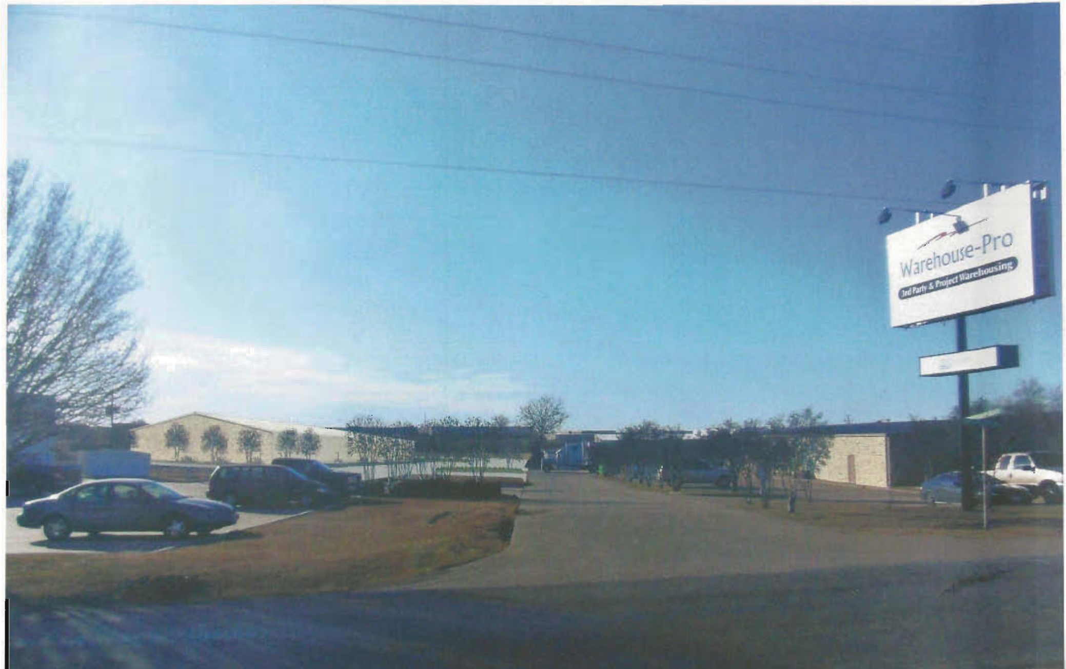
↑ NEW BLDG IN DISTANCE WITH STONE FRONT FACE ONLY RENDERING OF PROPOSED VIEW STONE ADDED TO EXISTING BLDG. ↑ NEAR I-30
