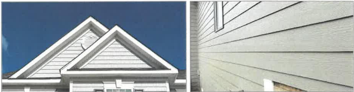
FIGURE 3: EXAMPLES OF HORIZONTAL LAP
