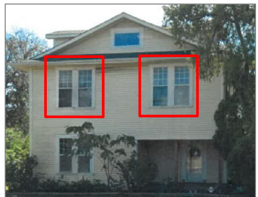
FIGURE 2: EXISTING WINDOWS TO BE REPLACED
