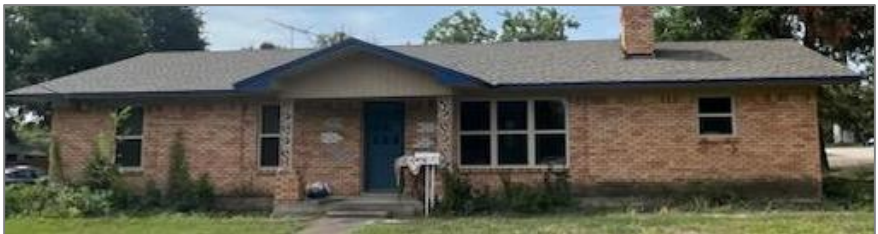
FIGURE 2: AUGUST 2, 2024. VIEW FROM E. RUSK STREET.
