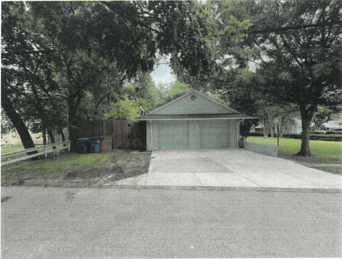
Picture 2: Existing driveway of 303 Williams off Fannin St.
