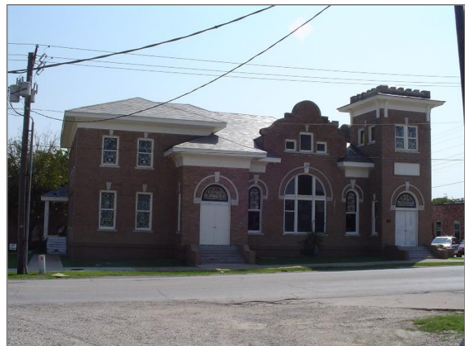
FIGURE 4: OLD METHODIST CHURCH AT 303 E. RUSK STREET
