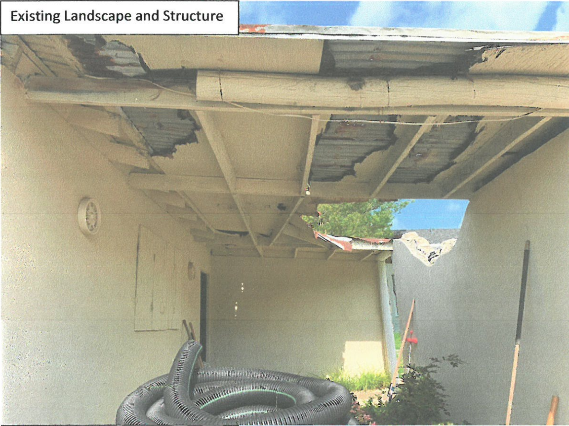
Existing Landscape and Structure
