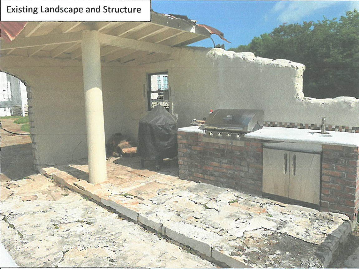
Existing Landscape and Structure
