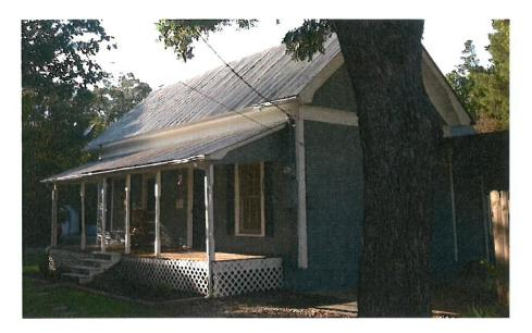
712 Hartman is not within the Rockwall Historic District, but a mere 2 blocks east. It currently has a standing seam metal roof of Galvanized Aluminum color.
