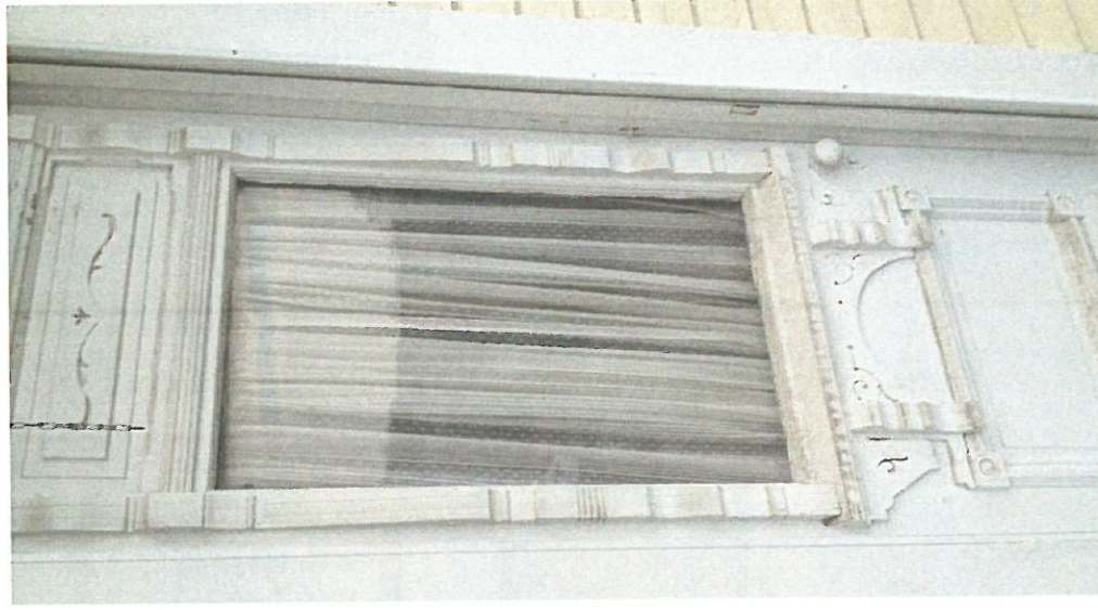
Original Upstairs Door
