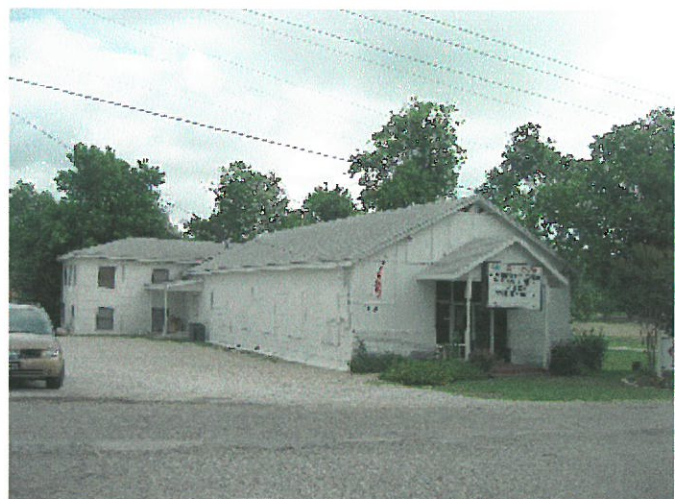
Current view from the west
