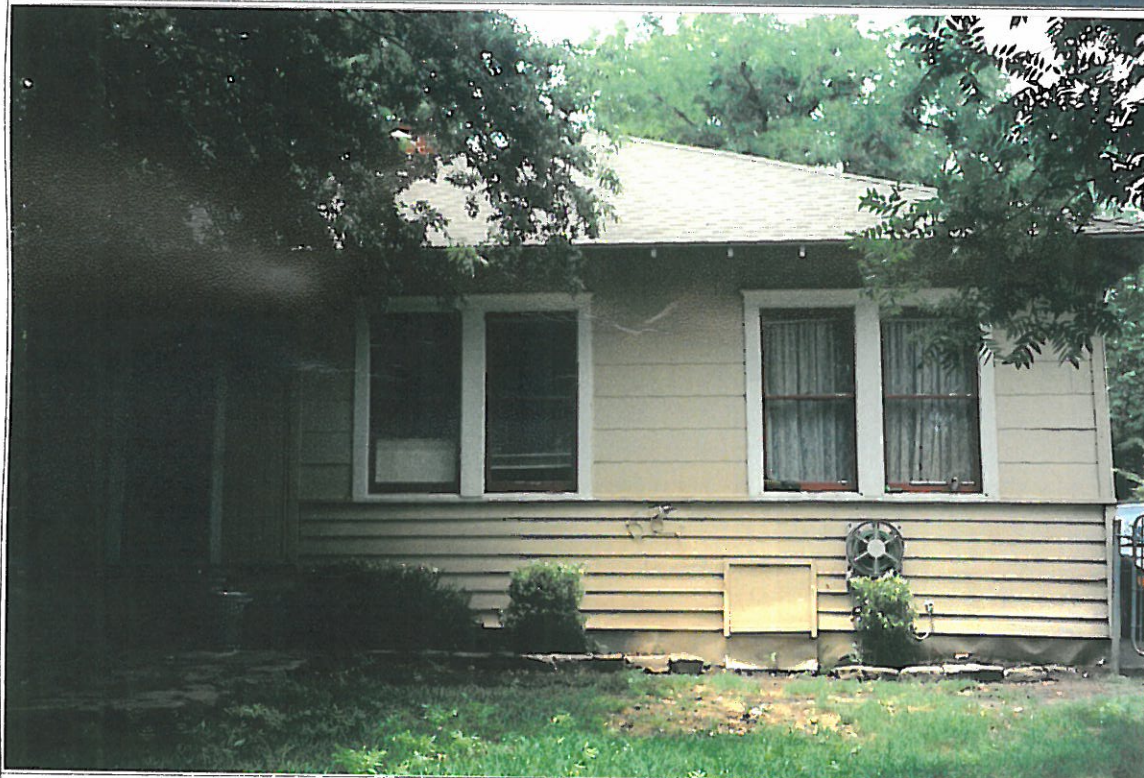
Rear View of Subject
