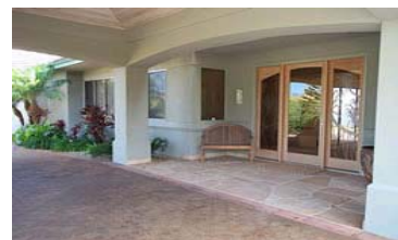
CARPORT TOP, PORTE-COCHERE BELOW
