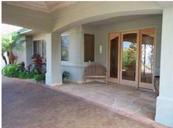
CARPORT TOP, PORTE-COCHERE BELOW
