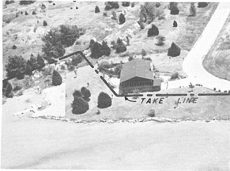
ENCROACHMENTS WITH HOUSE ON TAKE LINE
