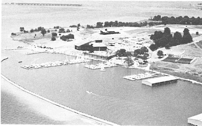
CHANDLER'S LANDING MARINA SHOWING EXPANSION SPACE BEHIND BREAKWATER
