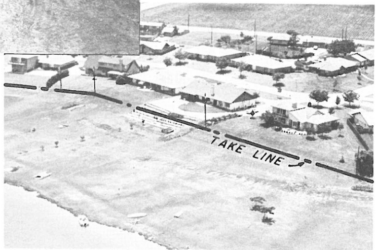
TERRACE CONSTRUCTION EXTENDING ONTO CITY OF DALLAS SHORE PROPERTY
