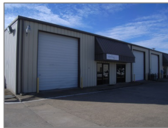
170: Multi-Tenant Building; 2010 Industrial Boulevard
