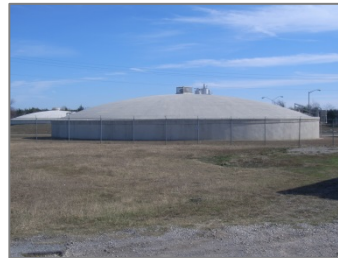
187: City of Rockwall Water Tank; 1308 & 1310 E. IH-30
