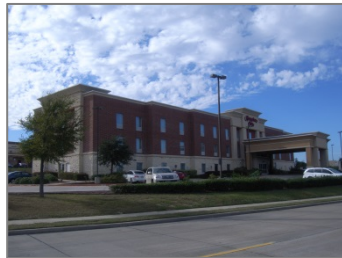
6: Hampton Inn; 1549 Laguna Drive
