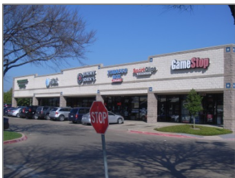
65: Steger Towne Crossing, Phase 1; 2779-2791 Ridge Road
