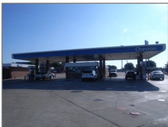
17: Chevron Gas Station; 600 E. IH-30
