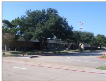
119: Rochell Elementary School; 899 Tubbs Road
