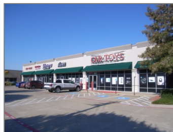
46: Shafer Plaza; 621-651 White Hills Drive
