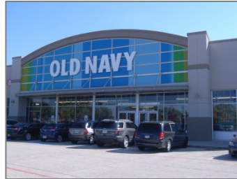
79: Market Center Shopping Center (Old Navy); 2875 Market Center Drive
