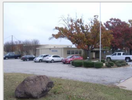
1 TXDOT Rockwall Maintenance Facility
