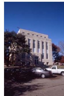
ROCKWALL COUNTY BUILDING IN THE DOWNTOWN SQUARE
