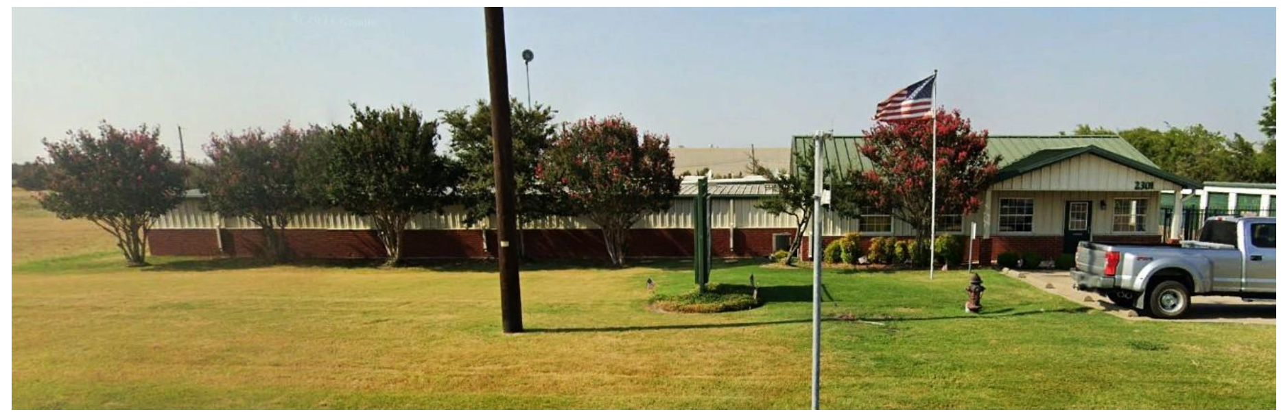
EXISTING HIGHWAY 276 FACADE
