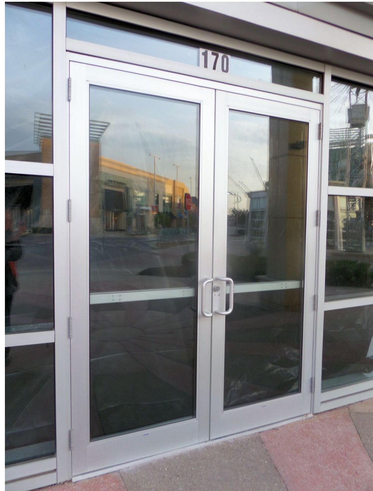
DOUBLE PANED GLASS PANEL SET IN 2" x 4 1/2" EXTRUDED ALUMINUM FRAME STOREFRONT LIGHT GRAY
