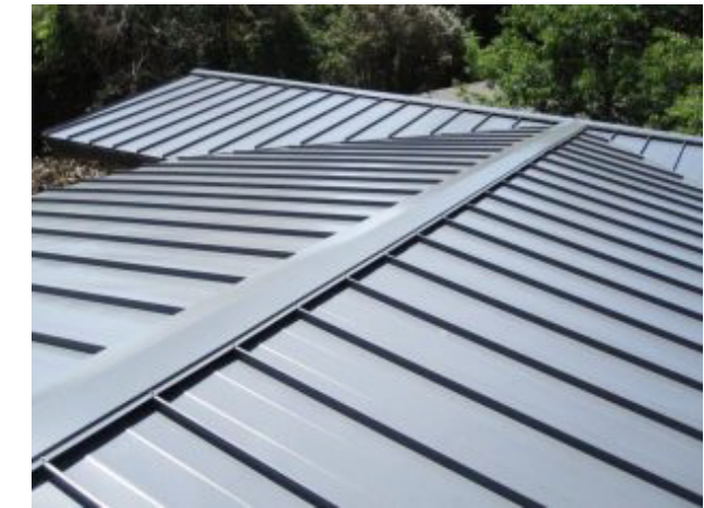
STANDING SEAM METAL ROOF SILVER METALLIC
