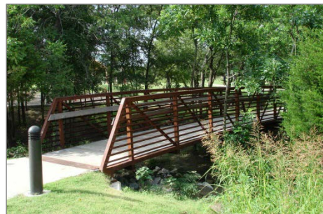
Bridge at Shores Park 2018: A pedestrian bridge connecting two (2) play areas and extending over a riparian area at Shores Park.
