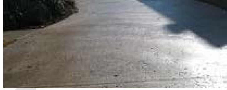
Rock Salt Finish Concrete
