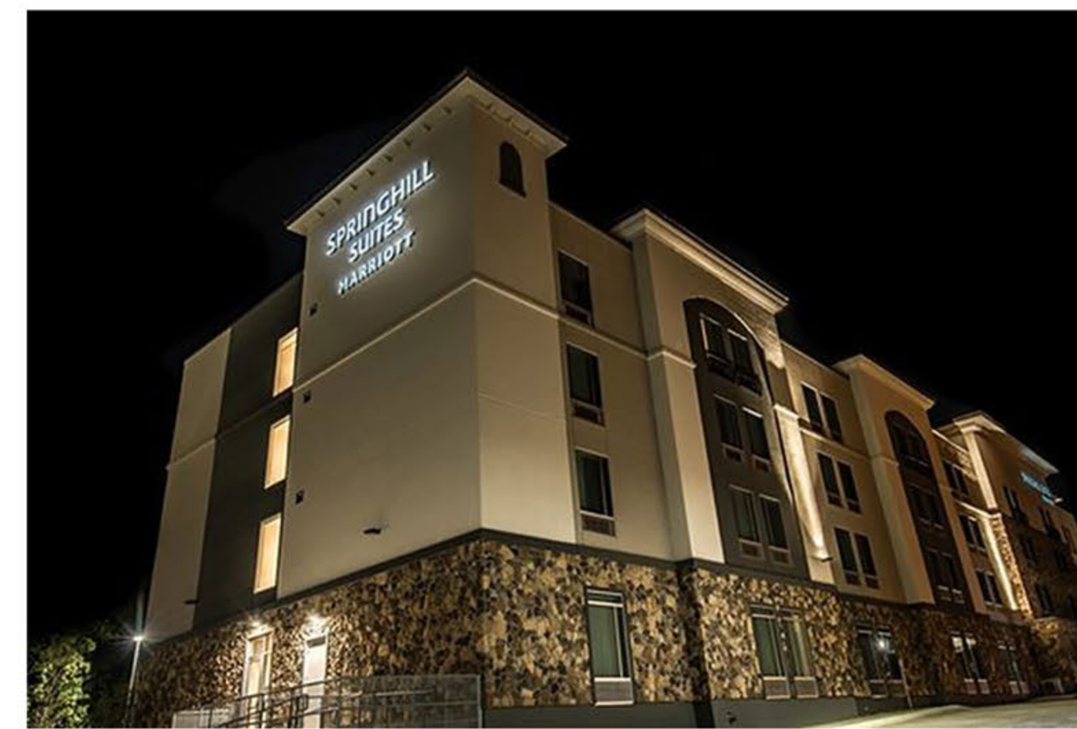
EXTERIOR MATERIALS: MASONRY BASE & EIFS with DRAINAGE SYSTEM
