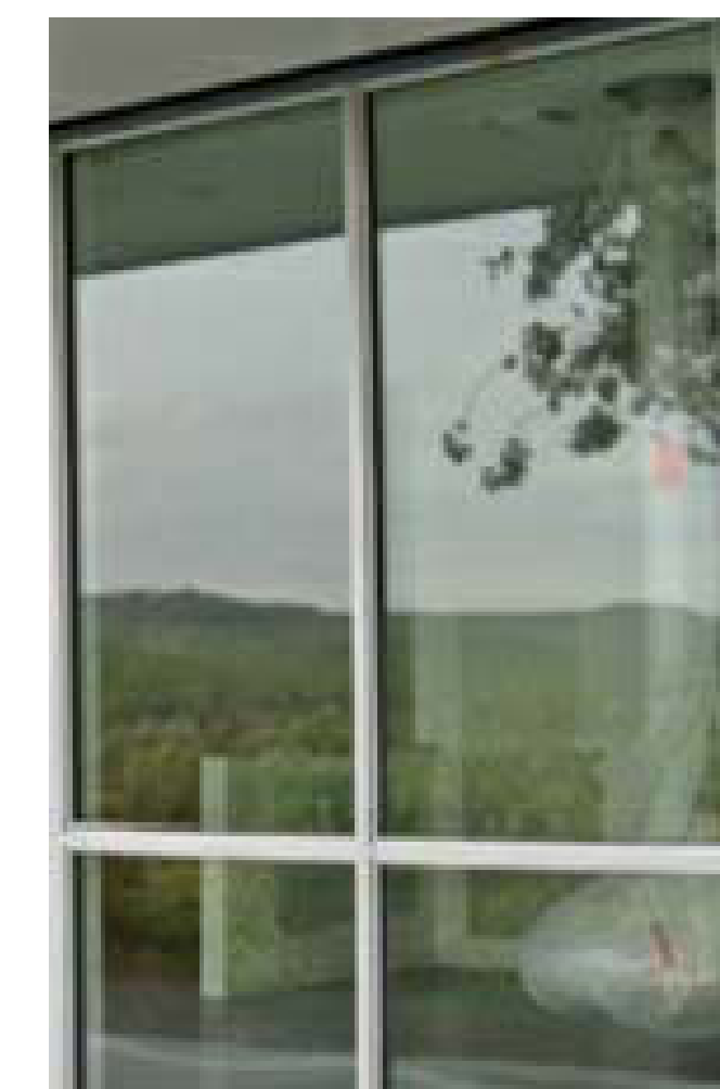
CLEAR ANODIZED ALUMINUM INSULATED GLAZING SYSTEM
