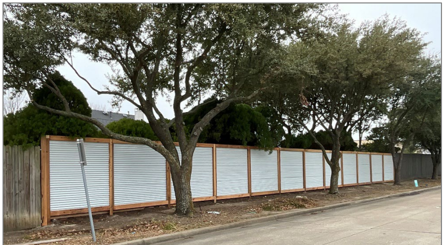
FIGURE 1: EXISTING FENCE - BUILT WITHOUT A PERMIT
