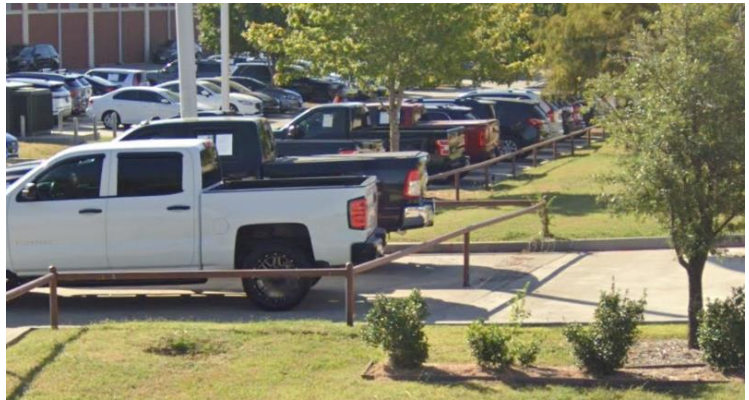
Figure 1: A photo taken from the IH-30 Frontage Road that depicts the existing pipe front yard fence.
