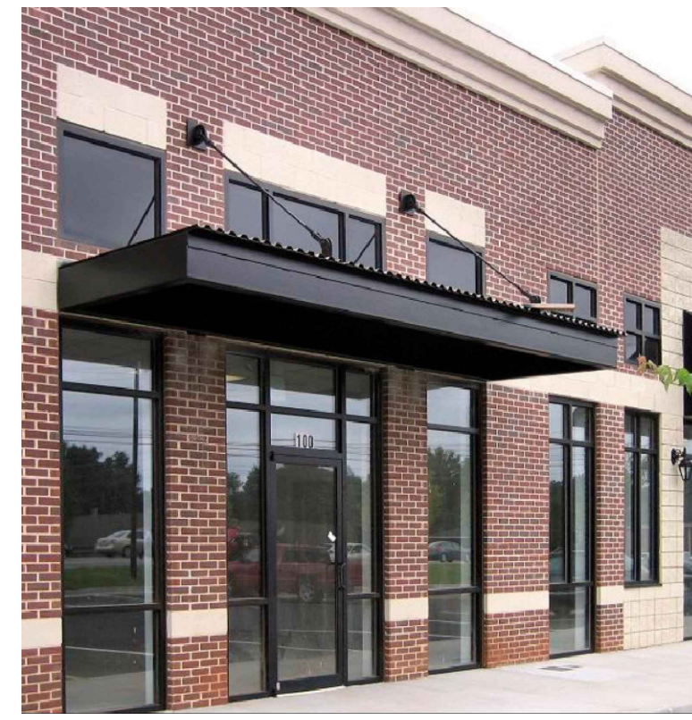
DARK BRONZE FRAMES, PARAPET CAP & CANOPY
