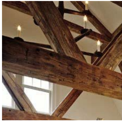
ST-1 Minwax Wood Finish 211 Provincial, 224 Special Walnut to accentuate knots and character in the wood. Topcoat: Clear Satin Polyurethane
