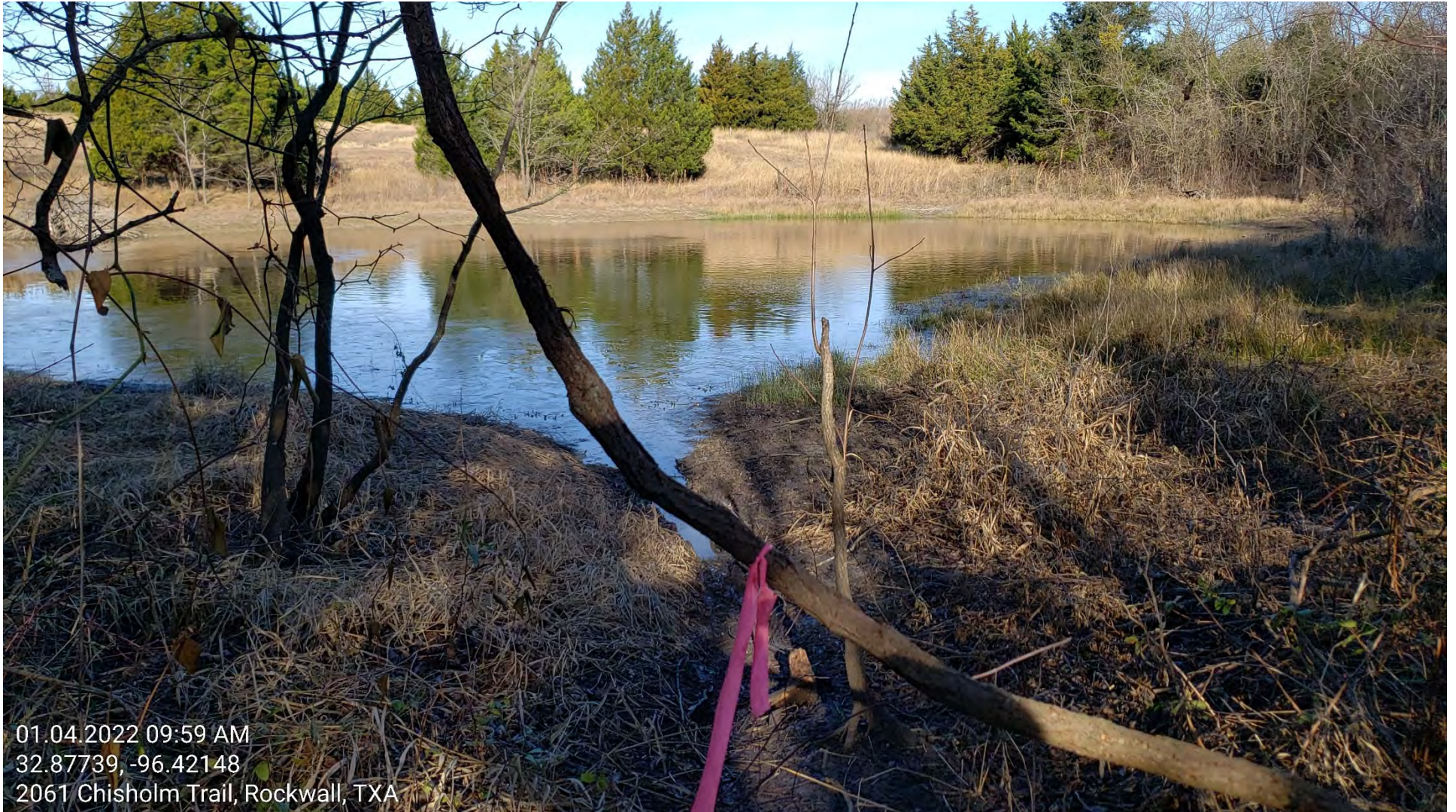
Photo 2: View of the pond from the southeast corner. The unfinished overflow channel in front, view partially covered by the tree branch.
