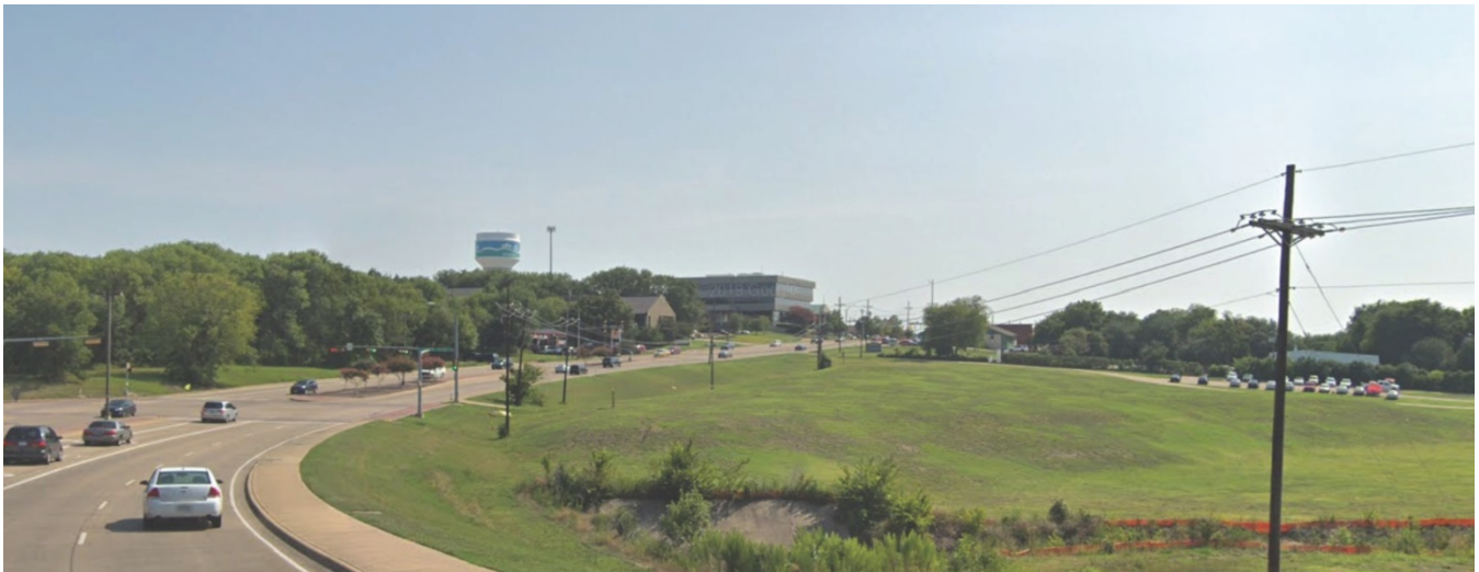
FIGURE 1: The subject property is depicted on the right-hand side of the above picture with Ridge Road being pictured on the left-hand side of the above picture.
