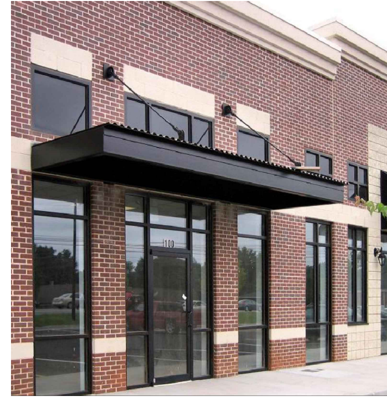
DARK BRONZE FRAMES, PARAPET CAP & CANOPY
