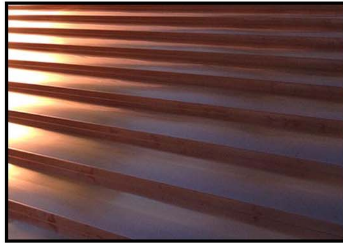
Copper Standing Seam Metal Roof
