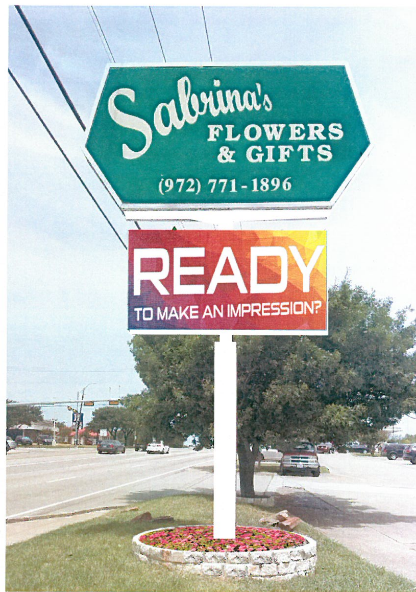
After: freshly painted pole and cabinets, new led lighting inside upper cabinet, retro-fit existing message board with led message center, update flower bed surround and landscape flower bed and yard
