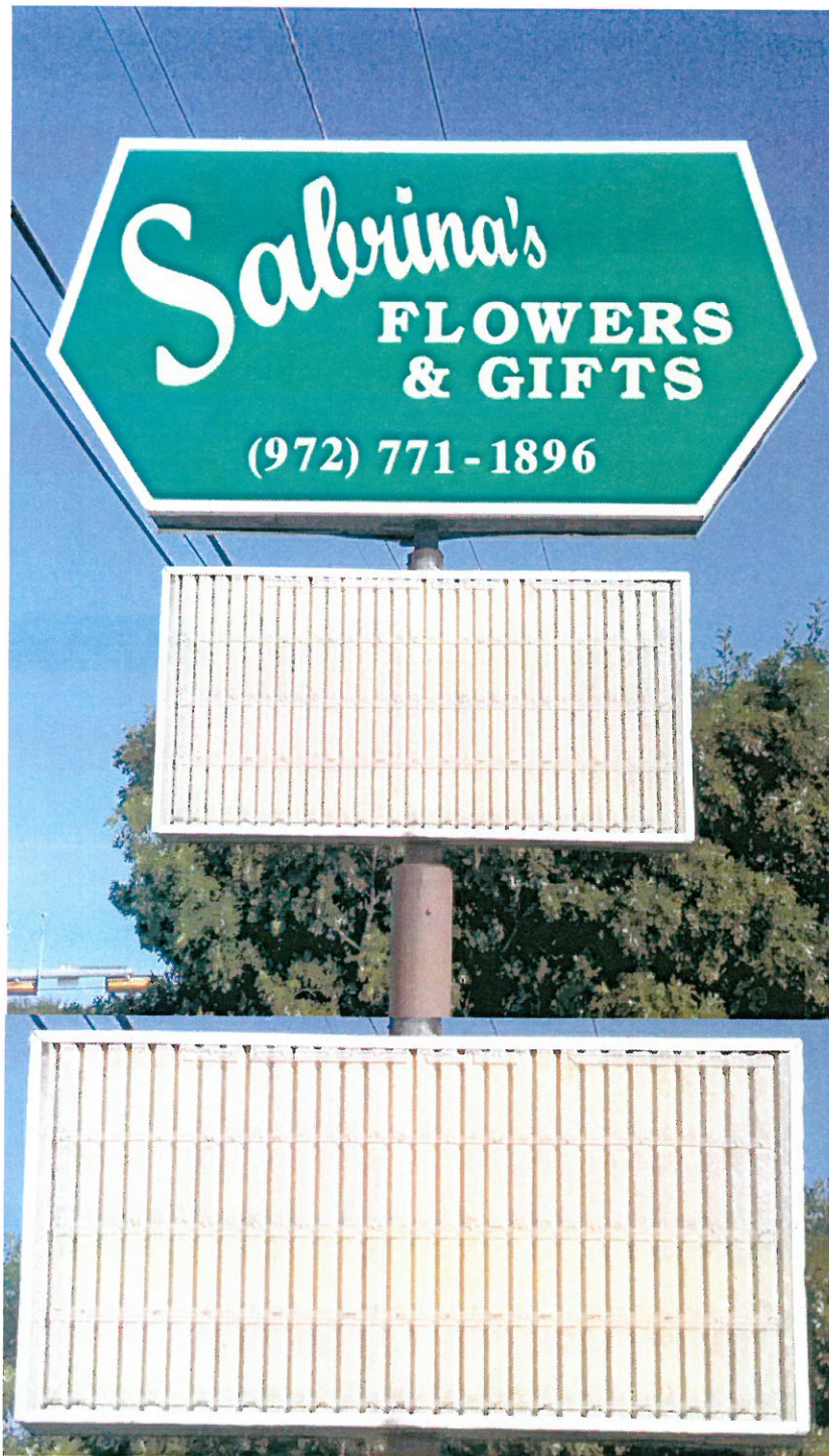
Before: corrugated acrylic message board that is rotted and yellowed, with multiple broken letter tracks.
