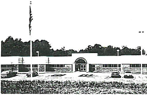
Michelin USA Tire Corp. Greenville, South Carolina Architect: CRS Serrine
