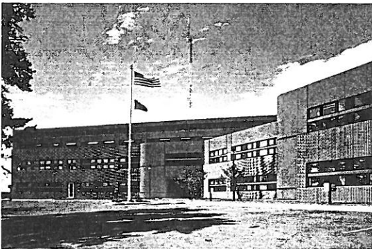
Burnett County Government Center Siron, Wisconsin Architect: Ozolins/D'Jock General Contractor: L. H. Sowles
