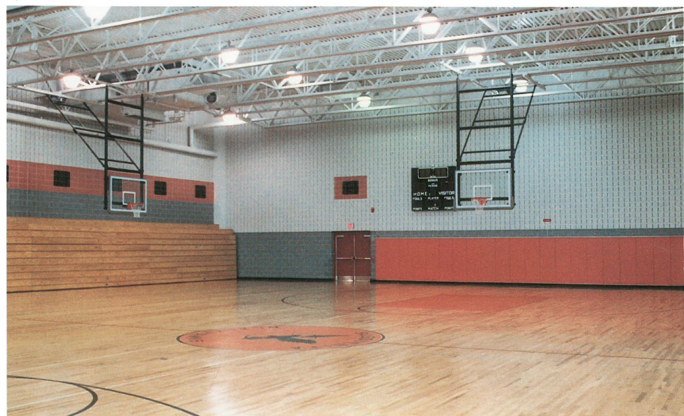
High School Gymnasium using ASTRA-GLAZE/ACOUSTA-WAL units.
