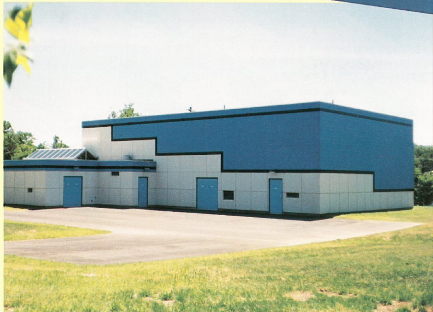
Wastewater Treatment Plant Harrison, Ohio.
