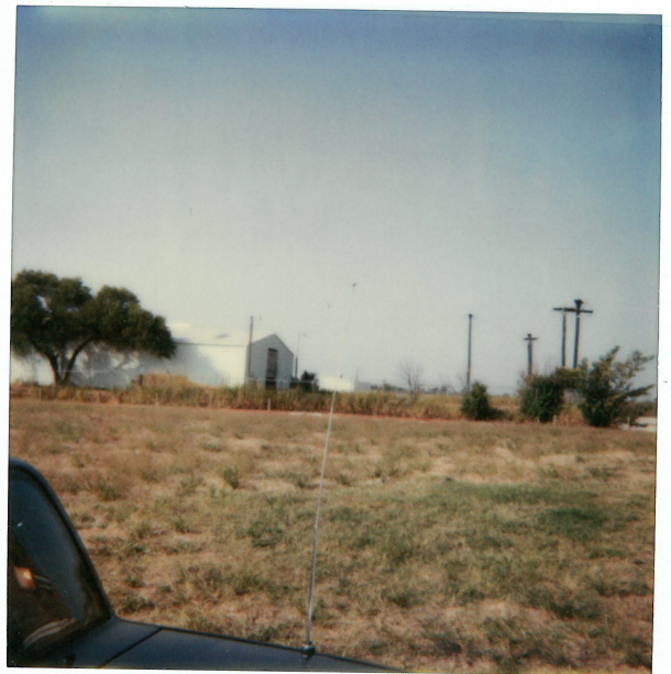
Rear view of building from Wal-Mart's south exit
